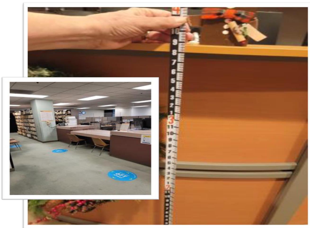
The inset photo shows an accessible counter at BSD-LDD Facility, Public Works headquarters.
