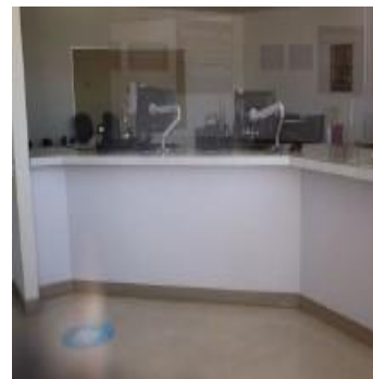
Counters in the top and right photos are mounted too high. Photo below shows counter height is 5" higher than the 34" maximum above the finished floor allowed.
