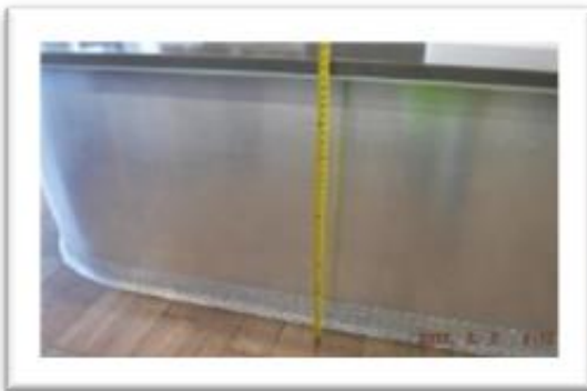
Photos above and to the right show counters that are mounted too high.
